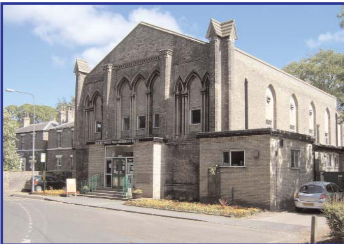
The picture shows the existing entrance to the Beverley War Memorial Hall which will become the ‘stage door’ entrance leading to a newly positioned stage. The main entrance to the building will be through Champney Road Gardens.
